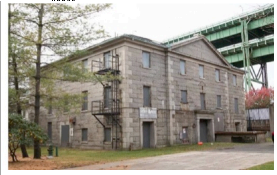
Existing Context - View of Ropewalk Head House
