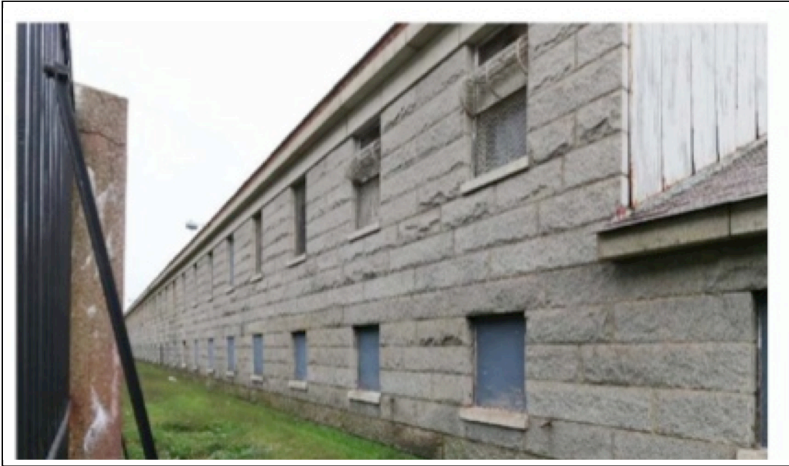
Existing Condition - View of West Elevation from Chelsea Street
