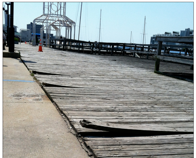
Broken planks on the Pier 8 boardwalk have been a chronic hazard for HarborWalk walkers, runners, wheel chairs, and carriages.
