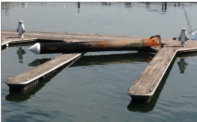
Piling down, an example of Pier 8's decline. Pilings have been falling for two years, most remaining unrepaired.
