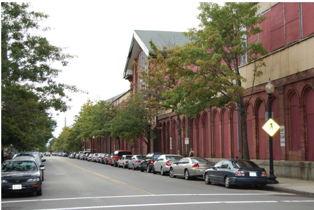
View of Chain Forge Shed from corner of 1 st Avenue & 13 th Street
