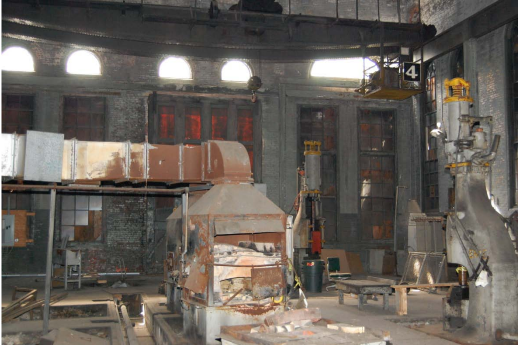
Interior View of Head House and Equipment
