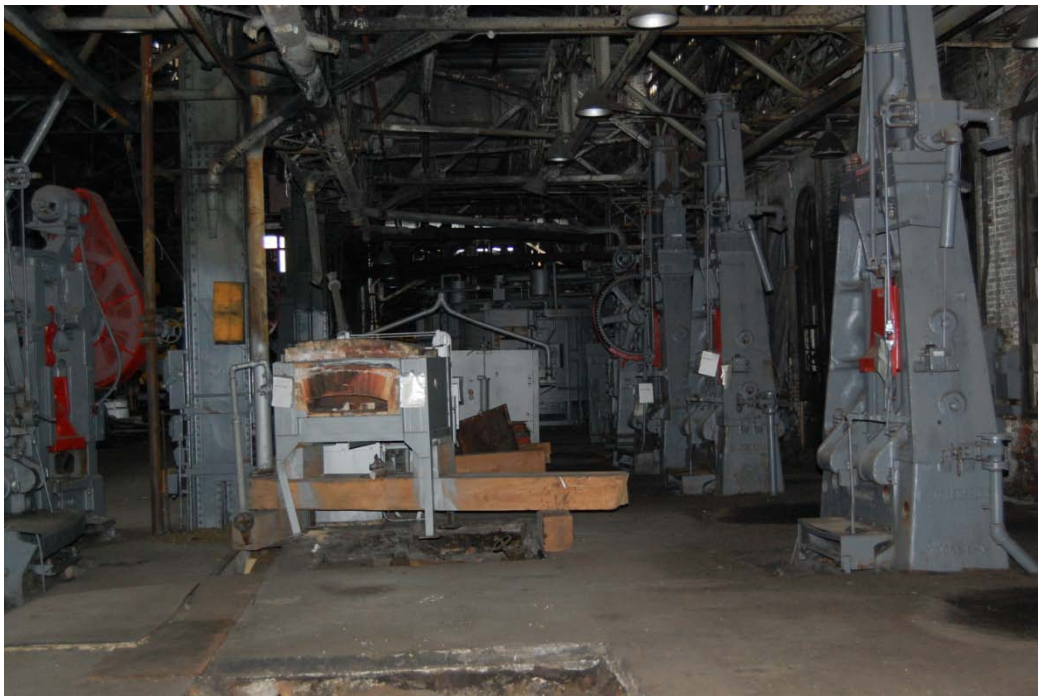
Interior View of Shed Building Machinery
