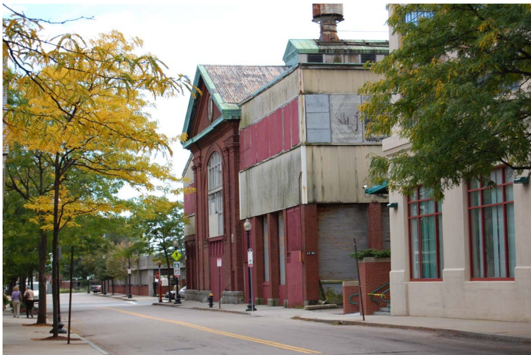
View of Chain Forge Shed from 13 th Street
